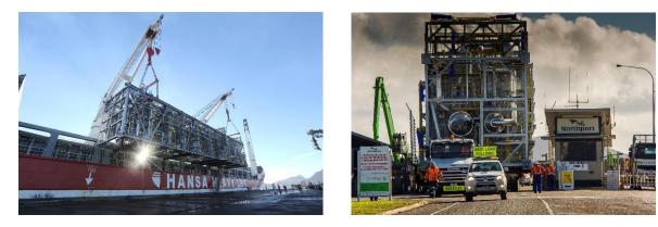
**Doubling up.** Modules for the Auckland ferry terminal pontoon weighing up to 165 tonnes were put into the water by Northport's two mobile harbour cranes and towed by tug to Auckland (below).
